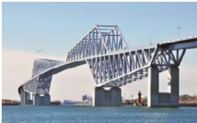
Fig. 1. Tokyo Gate Bridge [6]
