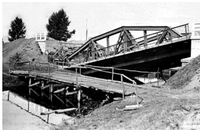
Fig. 4. Bridge damaged during the defence war in 1939 [13]
