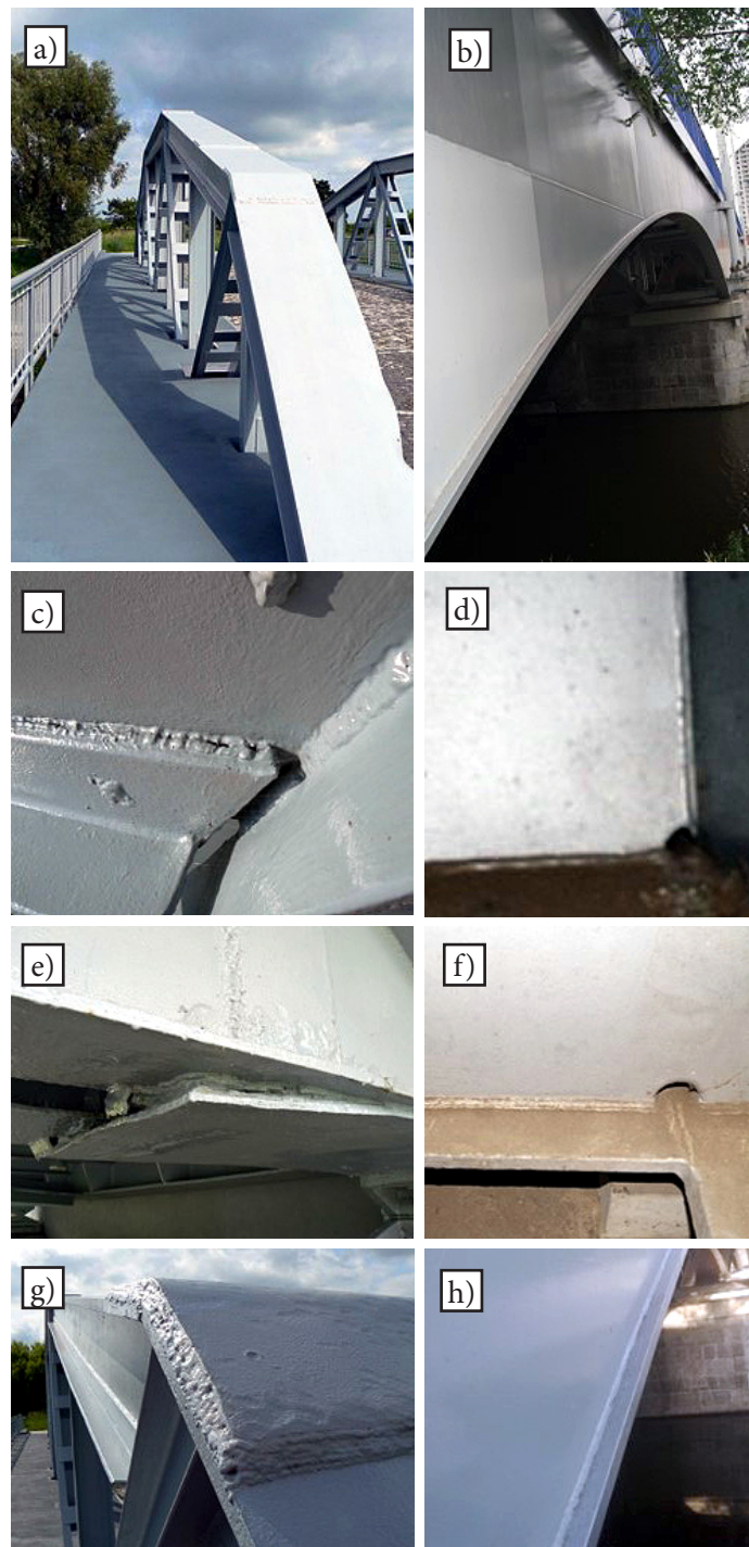
Fig. 10. Welded joints of load-carrying structures: the bridge over the river Słudwia in Maurzyce (a, c, e, g) and the footbridge on the Szczytnicki Bridge in Wrocław (b, d, f, h)
