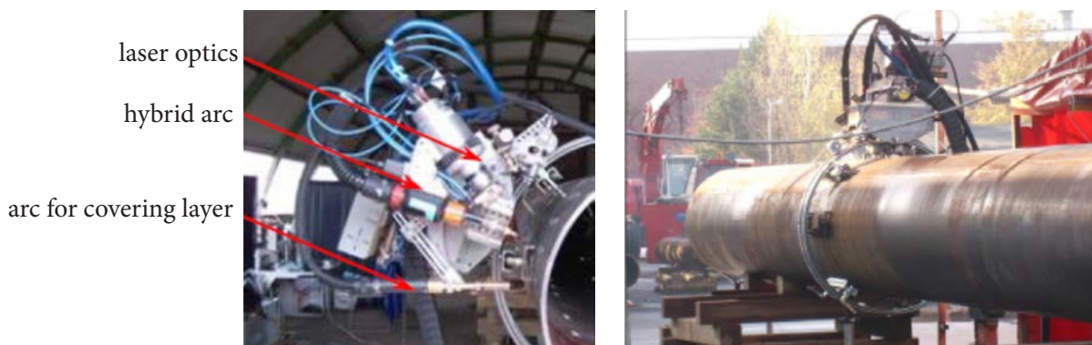
Fig. 6. Hybrid welding head with two arc welding torches (welding of the root and of the weld covering layer) and the whole test rig on the pipe
