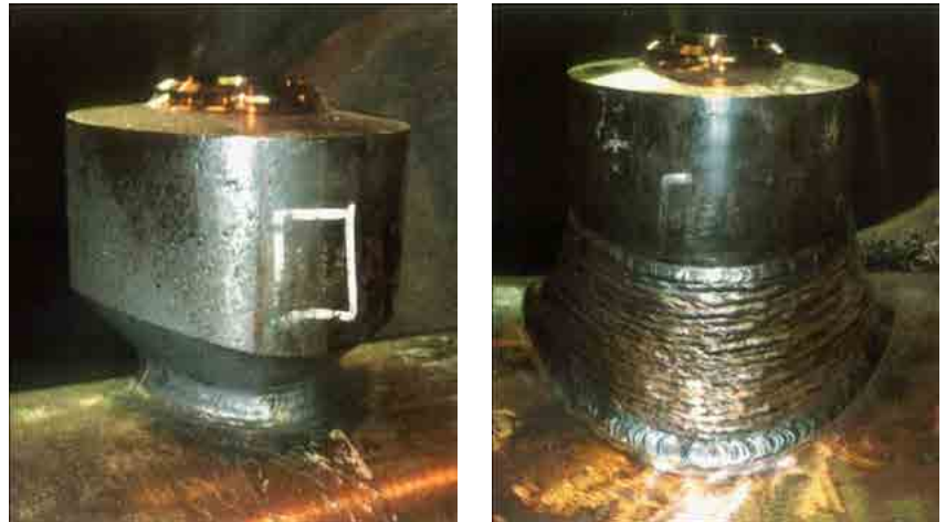
Fig. 3: Weld preparation and final weld in a pipe connection of a live-steam pipe of P91, welded with SMAW using Thermanit Chromo 9 V
