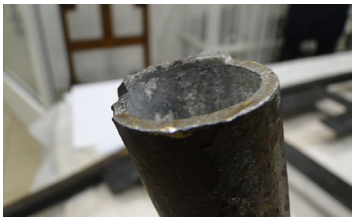
Fig. 6. End of the lower pipe (1DL acc. to Fig. 2) partially cut on along its circumference and then broken
