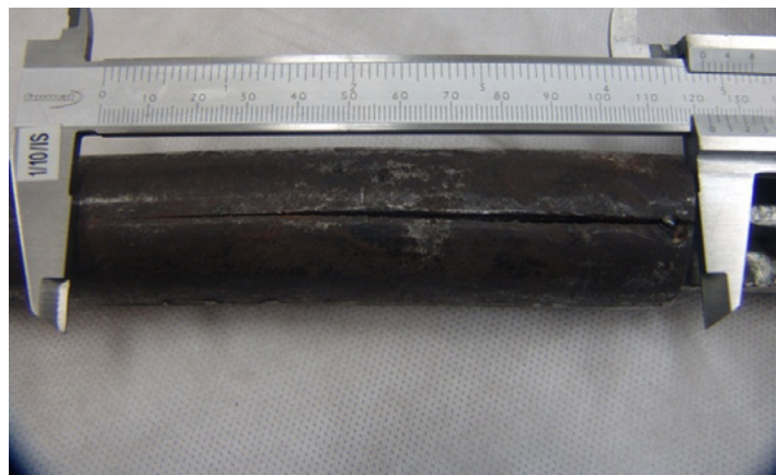
Fig. 7. 120 mm-long crack of lower pipe on section 1DL acc. to Fig. 2
