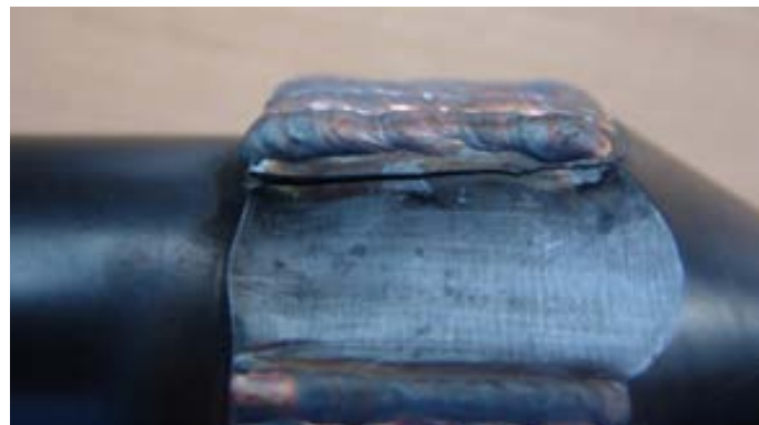
Fig. 6. Scaling of the surfaced layer of a punch made of steel 41CrAlMo7
