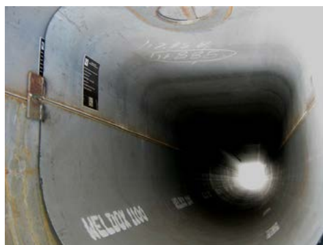
Fig. 2. HLA-welded segments of crane telescope pipe extension arm [25]
