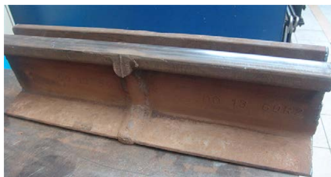
Fig. 2. Aluminothermic welded joints of 60R2 rails
