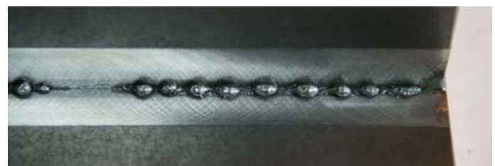
Fig. 5. Single-sided T-joint with excessive penetration on the root side
