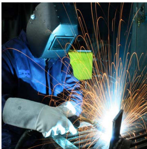
Conventional electric arc welding
