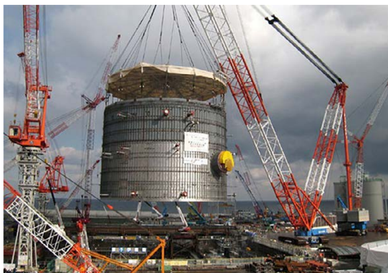
Fig. 3. Cylindrical fragment of an ABWR reactor liner manufactured by GE Hitachi [9]
