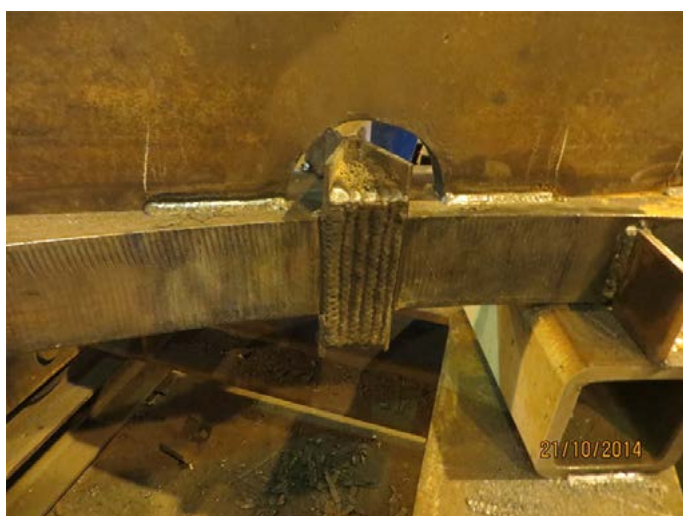
Fig. 5. Weld face from the internal side of a ring (also visible a clamp fixing the ring to the bed)
