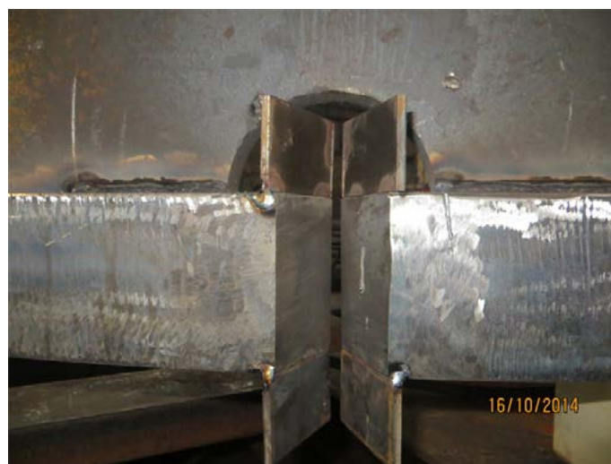
Fig. 3. Ring mounted on a welding station with run-on and run-off plates
