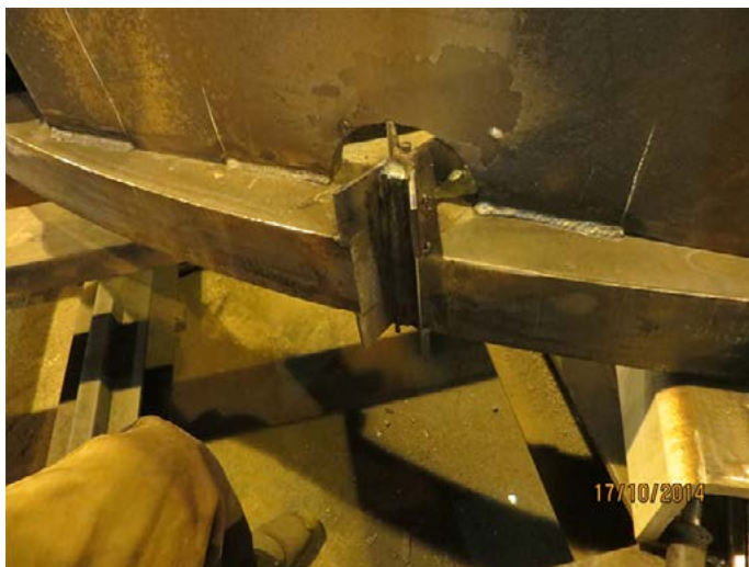
Fig. 4. Joint during welding
