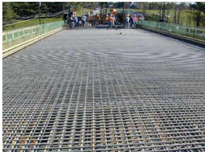
Fig. 9. Bridge in Morristown, Vermont; the reinforcement was made using GFRP composite rebars [21]
