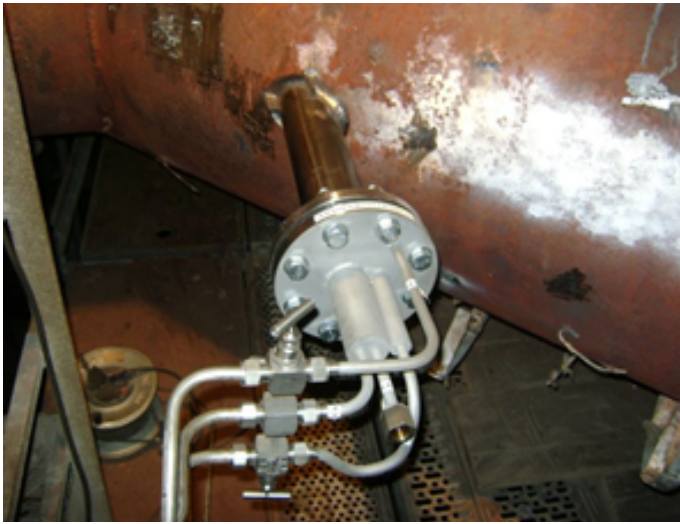
Fig. 6. Gas and liquid flow system with flowmeters containing laser welded impact pressure tubes
