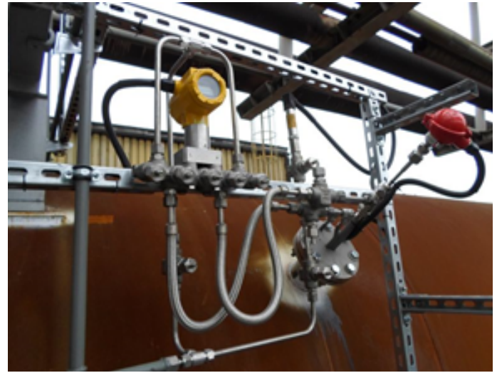
Fig. 6. Gas and liquid flow system with flowmeters containing laser welded impact pressure tubes
