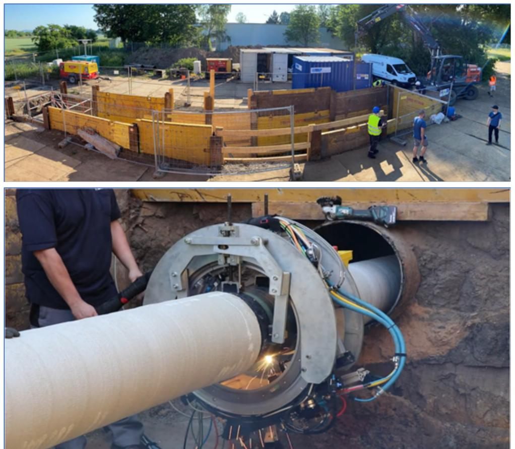
Fig. 8. Laser beam orbital welding performed on the construction site
